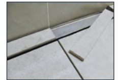
Invisible drainage system
